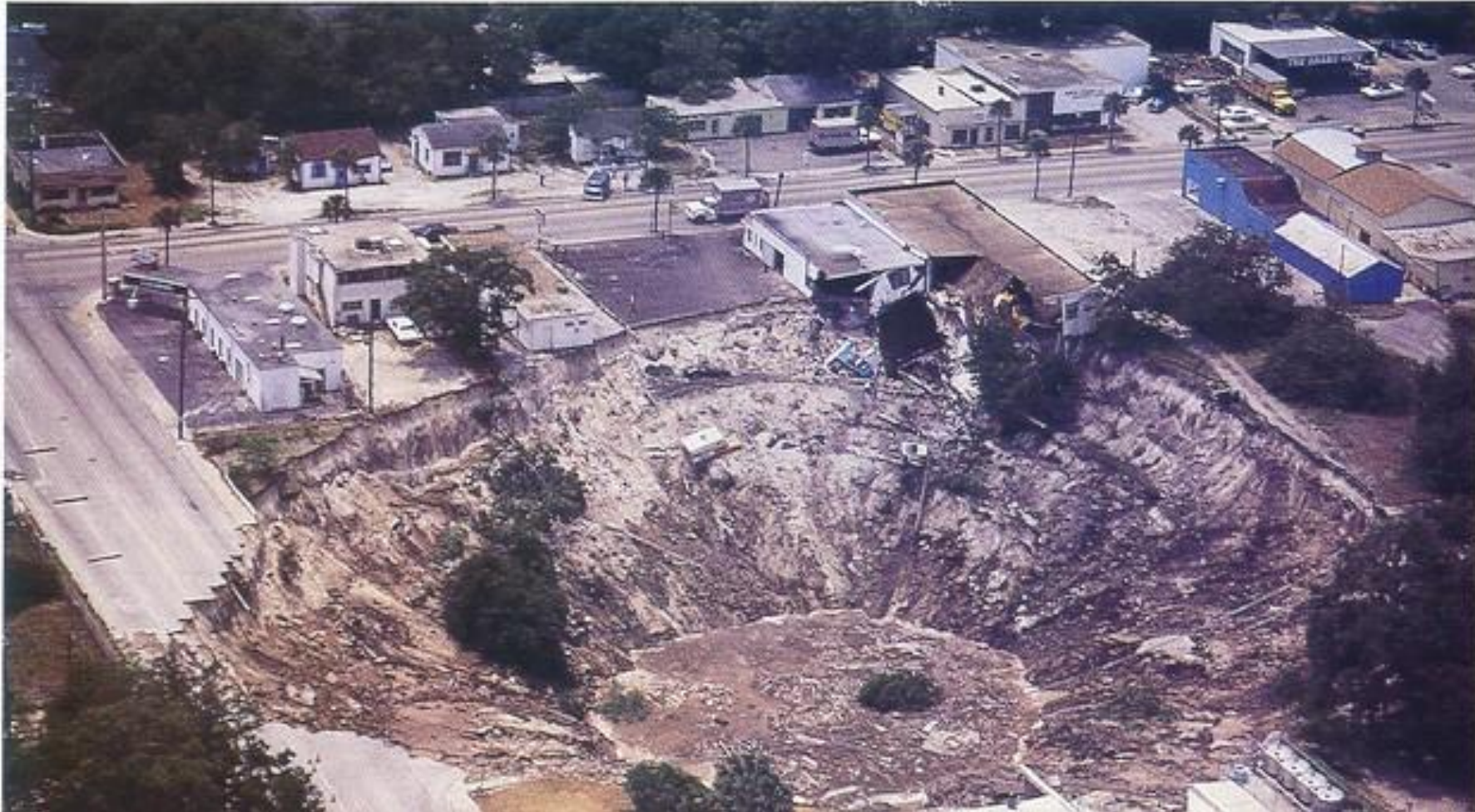
FIGURE 10.26. Most of a city block in Winter Park, Florida disappeared into a widening crater as this sinkhole formed in underlying carbonate bedrock.
