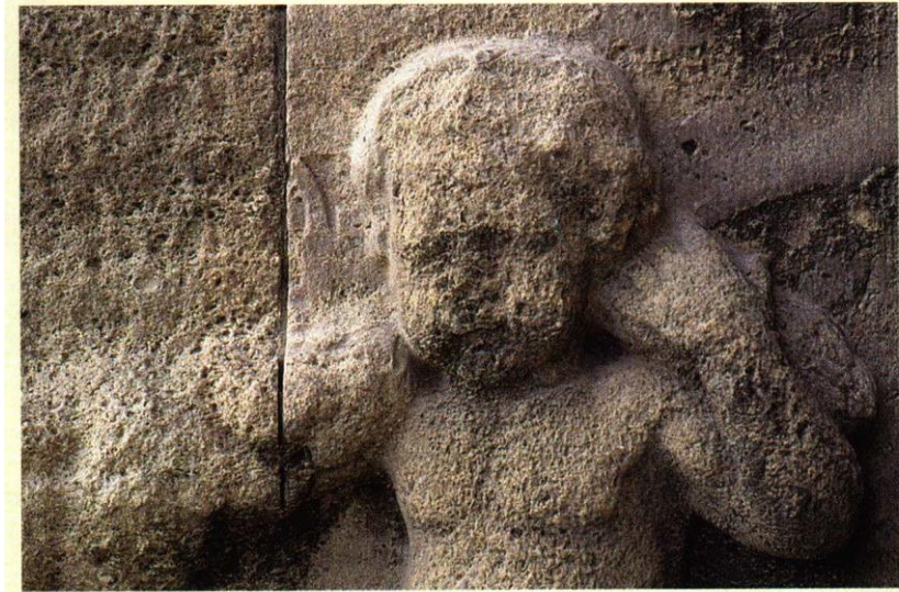
Figure 5.A Acid rain accelerates the chemical weathering of stone monuments and structures, including this building facade in Leipzig, Germany. (Photo by Doug Plummer)
